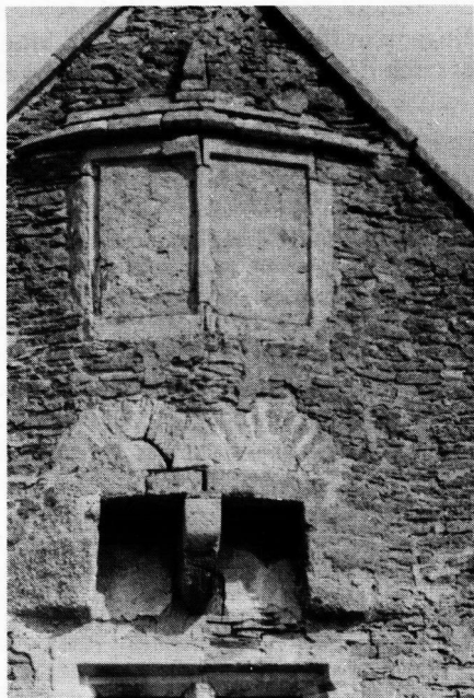
One of the oriel windows, roofed in stone and completed by an ornamental finial.
