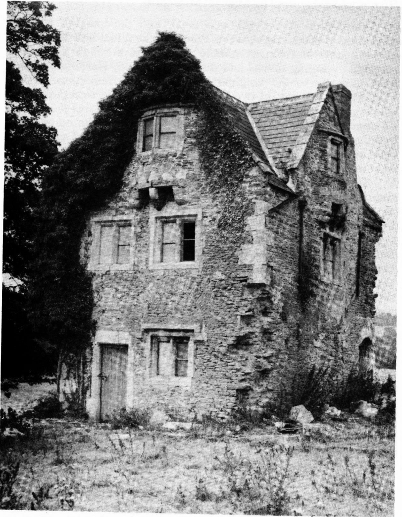
One of the architectural curiosities of Somerset: The Keeper's Lodge at Hardington , near Frome, now much dilapidated. A view from the south-west. Reproduced by kind permission of the Mendip Society.
